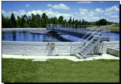
Hamilton • Hamilton STP 3 Clarifiers with Smith & Loveless HSA Suction Arm Mechanisms
