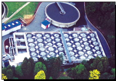
Tokoroa • Municipal STP FAST® Polishing Treatment System Duplex Gravity Filter Engineering Services
