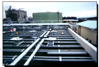
Winstone Pulp International Whitewater WWTP Turnkey/Design-Build FAST® Roughing Tower & Polishing Reactor Secondary Clarifier DAF
