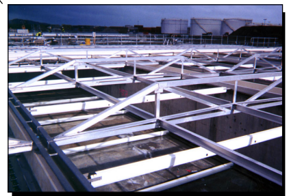
Wellington-Hutt • Lower Hutt WWTP 4 FinnChain® Primary Clarifiers completed with S&L Scum Baffles
