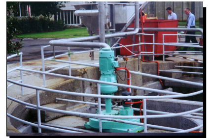
Rotorua • Rotorua STP 2 PISTA® Grit Chambers 2 PISTA® Turbo Grit Pump 2 PISTA® Grit Concentrator 2 PISTA® Grit Screw Classifier Complete Headworks Upgrade
