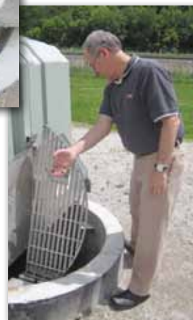
Above: view of an open wet well grate. Right: As a pump station operator demonstrates, accessing a wet well with fall protection is as easy as pulling the handle.
