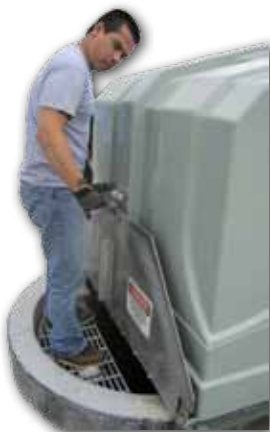
Above: view of an open wet well grate. Right: As a pump station operator demonstrates, accessing a wet well with fall protection is as easy as pulling the handle.
