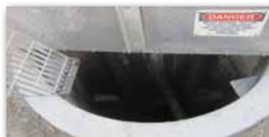
Above: view of an open wet well grate. Right: As a pump station operator demonstrates, accessing a wet well with fall protection is as easy as pulling the handle.
