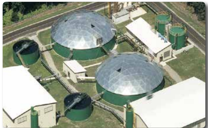
(Pictures above) At this field-erection site, Smith & Loveless coordinated its work with other contractors and crews on-site. They all meet their critical deadline—complete field-erection, installation and start-up in less than three months.
