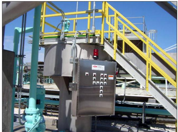
When a glass bottler subsidiary of a major U.S. brewer sought to reduce their hauling costs and hassles associated with its industrial washdown water, they contacted Smith & Loveless for tangible solutions. Specifically, the company wanted to recover the cullet (broken glass chips) accumulated in its large production process and prevent difficult-to-handle sludges, which had become cost-prohibitive. Because this Texas bottle manufacturer produces more than
