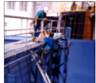
S&L provided a Model R OXIGEST Wastewater Treatment System complete with treatment zones, clarifier and denitrification processing in a single tank to aerobically polish high strength industrial wastewater. Fine bubble diffusion (above left) is employed for efficient oxygen transfer. The S&L field erection crew (right) puts the finishing touches on the plant.
