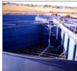
S&L provided a Model R OXIGEST Wastewater Treatment System complete with treatment zones, clarifier and denitrification processing in a single tank to aerobically polish high strength industrial wastewater. Fine bubble diffusion (above left) is employed for efficient oxygen transfer. The S&L field erection crew (right) puts the finishing touches on the plant.
