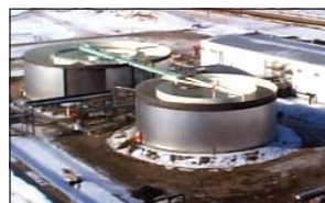
Alberta - Industrial Wastewater Model R OXIGEST® & Spill/EQ Tank 2,900 m 3 /d
