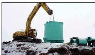
British Columbia - Municipal Collection Custom Series Underground Pump Station 100 lps
